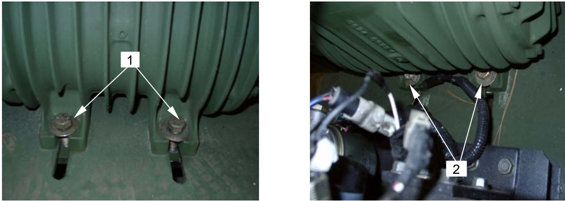
Figure 6. Removing Vacuum Pump Mounting Bolts
